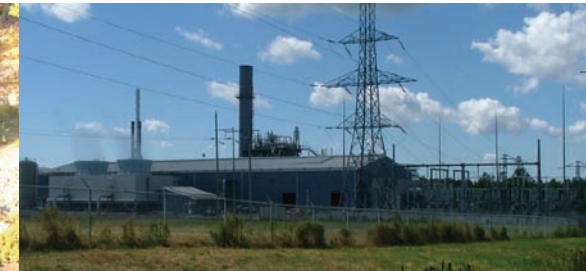
This cogeneration plant near Kingston uses a waste energy recycling process to produce both electricity and industrial steam for adjacent industries.
