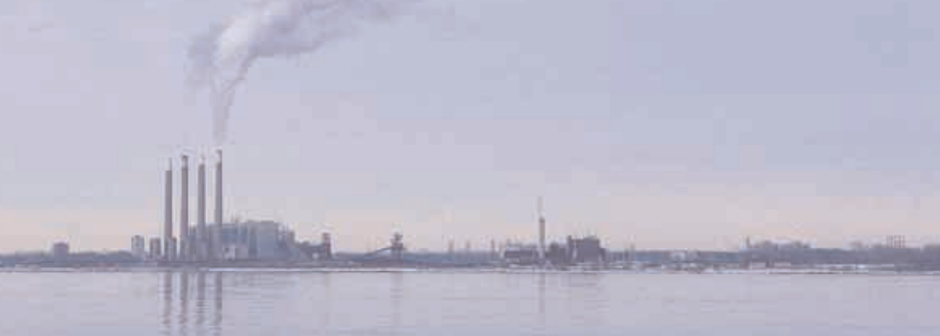
Cause and effect: (left) Lakeview Generating Station is a Toronto-area coal-fired electricity plant that releases CO 2 .
