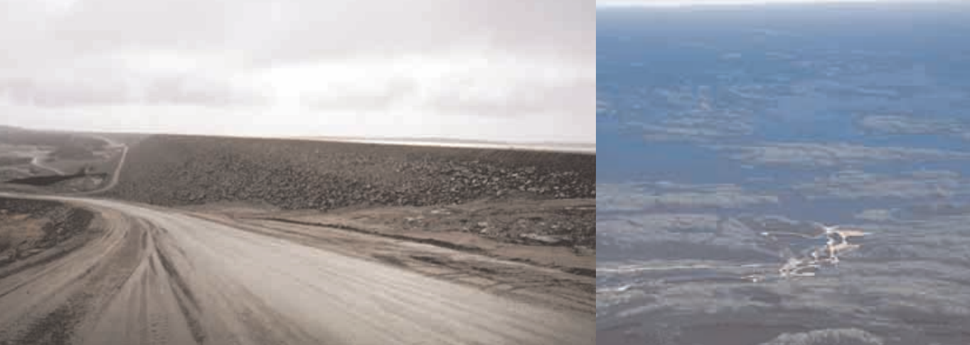
(Far left The James Bay hydro-electric development and the Robertson Lake hydro-electric development (left) in Quebec.
